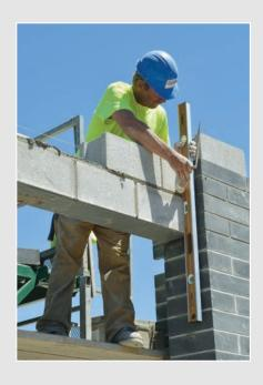
For the mason, Johnson offers dot and line lasers for alignment and masonry-specific levels such as our EZ-Clean™ bamboo levels – available with either top read block vials for working above the level, or curved vials for smoother bubble travel.
