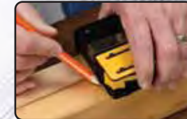
3" Layout for Double Framing Members
