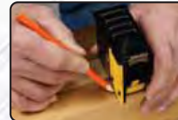
1-1/2" Layout for Single Framing Members
